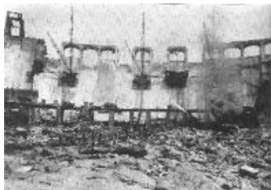
Construction of Martin Dam - Approx 1925
